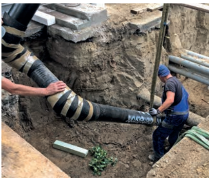
Laying the BRUGG-STAMANT® safety pipe with sure instinct
