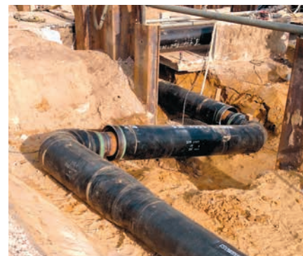
BRUGG-STAMANT® Safety Pipe with expansion element
