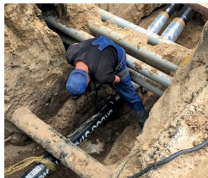
Professional connection to the existing BRUGG-STAMANT® Safety pipeline
